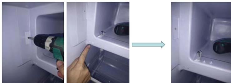
Step 1: remove the inner door block & screw hole plug.
